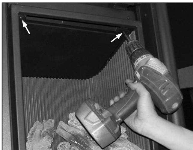
Figure 12: Firebox Baffle Screws Removal.
